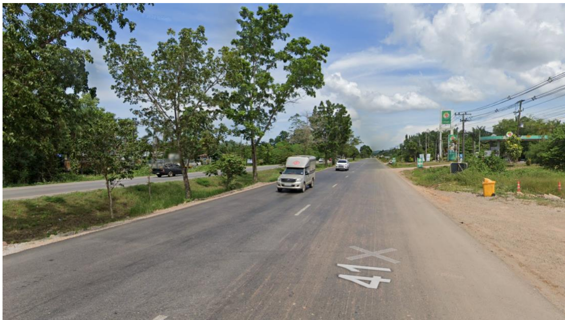
Start points. A single road section (Google Streetview image).
