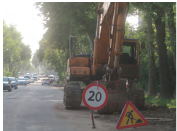
Regulatory speed restriction signs may also be used for temporary use such as at road works or where an emergency situation demands traffic to slow (photo by Phil Jordan).
