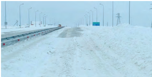
Motorway in Kazakhstan with median barriers, yet with elevated risk of serious crash due to snow (photo by Soames Job).
