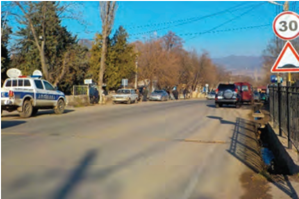
Road with a 30 km/h speed limit in Georgia combined with a speed hump (photo by Soames Job).
