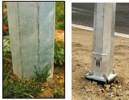
Impact absorbent lighting columns are suited to low speed areas (less than 80km/h) where there may be more pedestrians and more parking nearby.
