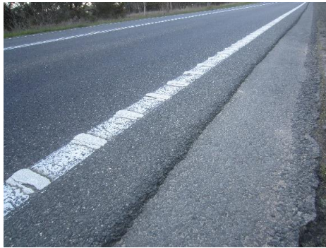
Tactile edge lines have been proven to reduce run-off-road incidents. They are best used in combination with sealed shoulders.
