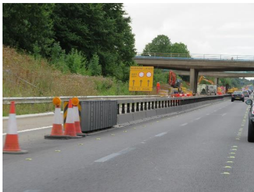
Some impact attenuators are designed to be used in narrow areas at road work sites.
