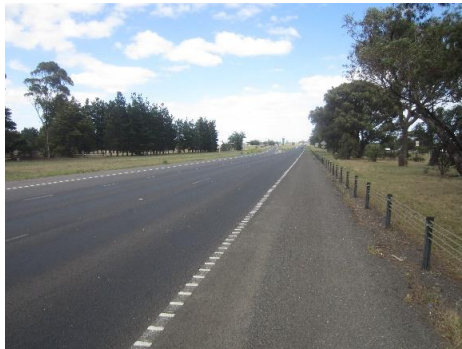
Tactile edge lines alert fatigued or distracted drivers to the fact they are drifting off the highway.
