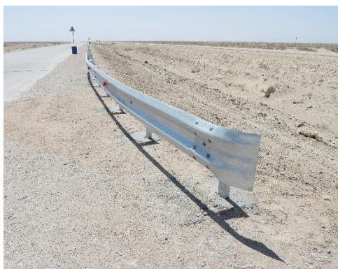
"Fish tail" terminals present a spearing risk and should not be used on CAREC highways.
