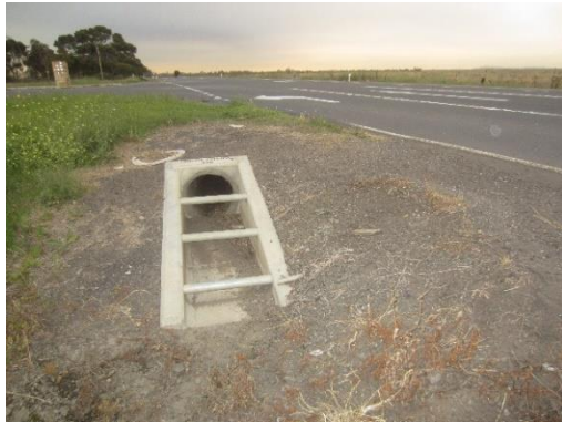
A Type 1 drivable end wall is suitable for shielding the ends of pipes parallel to the road.
