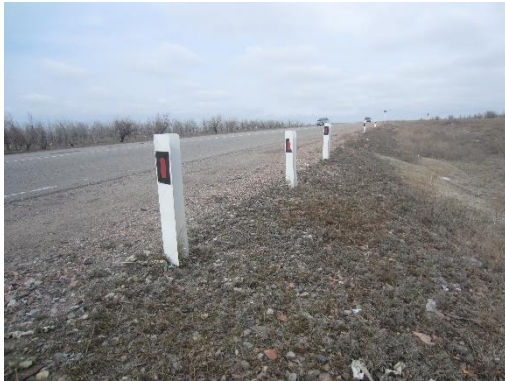
Lightweight steel guide posts can provide useful delineation. Large areas of reflective material are an important element of useful guide posts.
