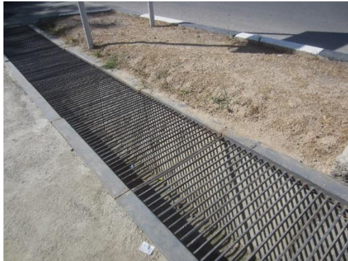
Covering drains that are within the clear zone can give a smooth drivable and more forgiving area.
