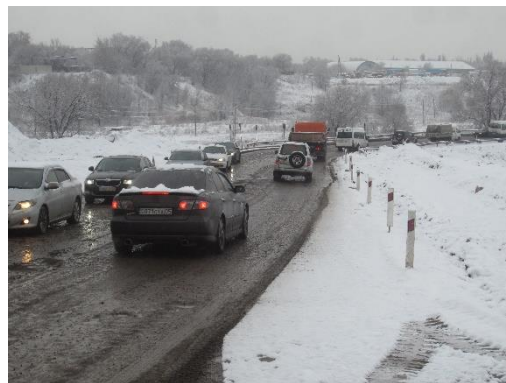
CAREC highways encounter some tough weather conditions. Guide posts are essential to guide drivers and to assist them to remain on the road in snow
