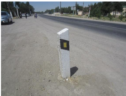
Reinforced concrete guide posts are roadside hazards. They should not be used on CAREC roads.
