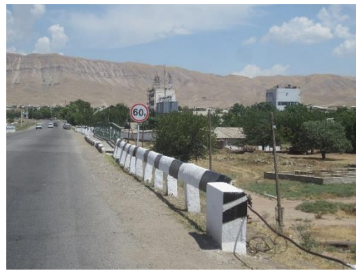
Concrete blocks and concrete barriers like this are roadside hazards. At best they offer some limited delineation only.
