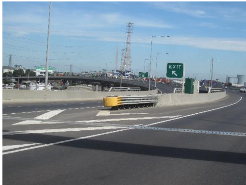
Impact attenuators are well suited to shielding rigid barrier ends in confined and heavily trafficked locations
