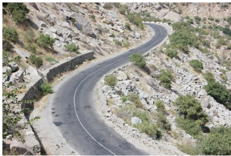
The highway is a 2 lane 2-way highway passing through hilly terrain. It has generous geometry and is subject to a national speed limit of 100km/h.
