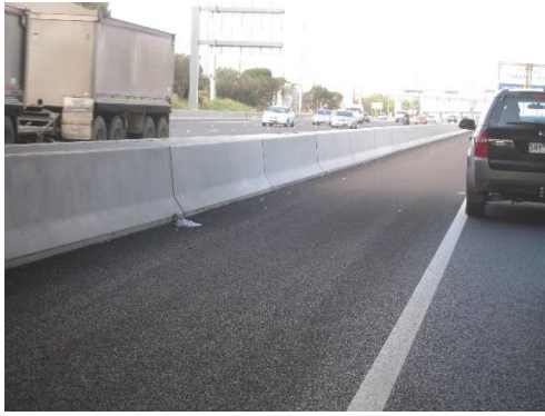
Rigid barriers allow high containment levels to be attained within narrow cross sections, while (in this photo) still providing sufficient space for a wide inner shoulder.
