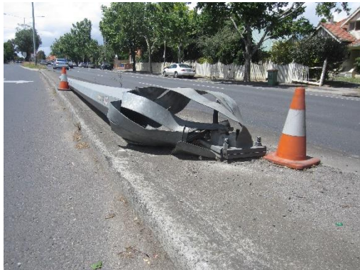
Impact absorbent poles (such as this one which has been struck) help to minimize injuries to the vehicle occupants.
