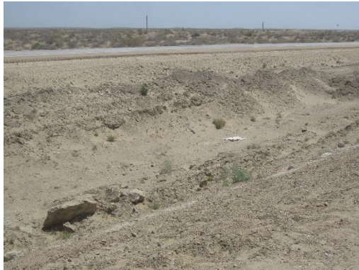
The highway has been designed to high geometric standards. The median has been graded for natural drainage in the desert environment.
