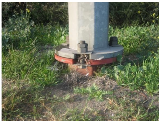
Slip based lighting columns are suitable for use in high speed areas (80km/h and above) where there are few pedestrians and little parking.
