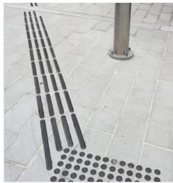
Figure 30: Discrete TGSIs (individual studs)
