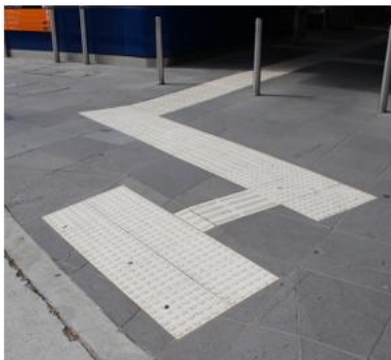
Figure 29: Integrated TGSIs (tiles)
