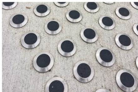
Figure 31: Discrete TGSIs (individual studs - composite / two tone)
