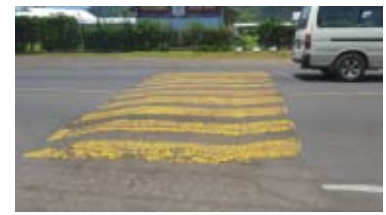
Photo 3 – Pedestrian Crossing with zig zag yellow crossing bars on raised platform – LTA in house design
