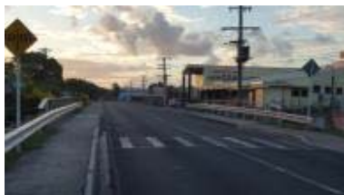
Photo 1 – Pedestrian Crossing with parallel white crossing bars on flat surface - designed and constructed using Austroads & NZTA Stds, WB funded project
